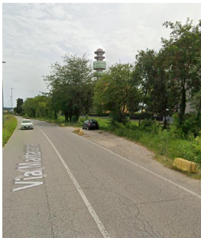
La zona Telecom in Via Mattarana
